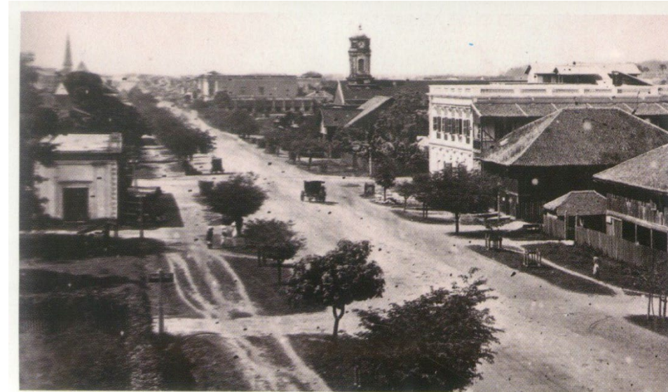
Merchant Street circa 1865 (photo: Bentley & Jackson). Looking west, Trinity Church spire left, old Catholic Church right.
